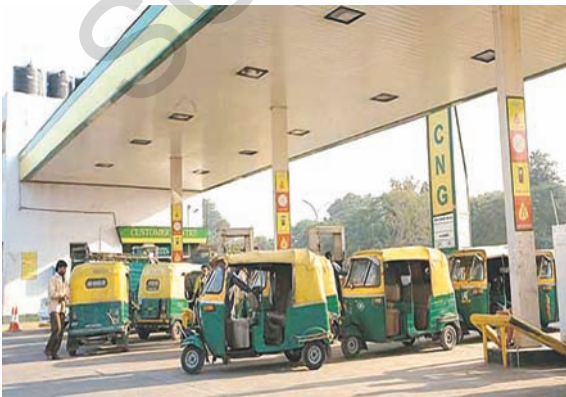
Fig - 3: CNG gas filling station
